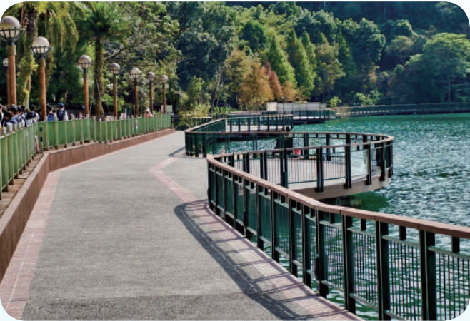
伊達邵至纜車站自行車道串聯工程 Ita Thao to Cable Car Station Bikeway Connection Project
