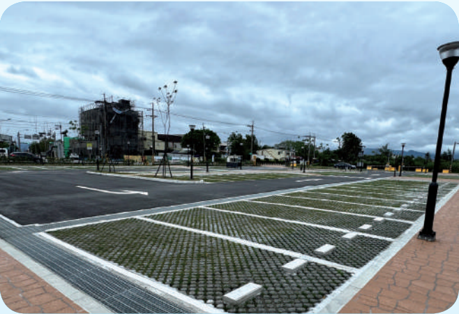
壯圍沙丘生態園區周邊設施優化工程 Zhuangwei Dune Ecological Park Peripheral Facility Optimization Project
