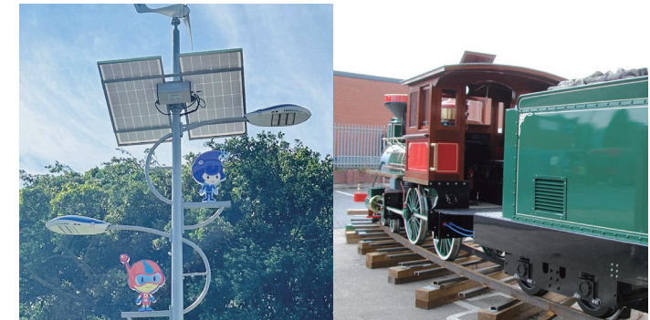
優質化計畫補助 - 左：小叮嚀科學主題樂園風光雙軌儲能式 LED 路燈 右：九族文化村小火車柴油引擎電動化 Quality Enhancement Subsidies - Left : Dual-track wind-solar energy-storage LED streetlights at Little Ding-Dong Science Theme Park; Right : diesel-to-electric conversion of the miniature train at the Formosan Aboriginal Culture Village
