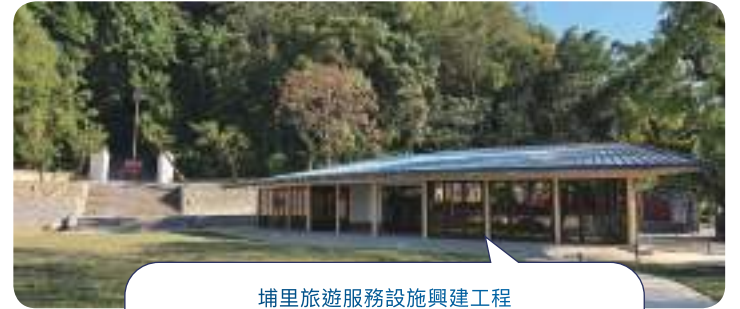
埔里旅遊服務設施興建工程 Puli Tourism Service Facilities Construction Project
