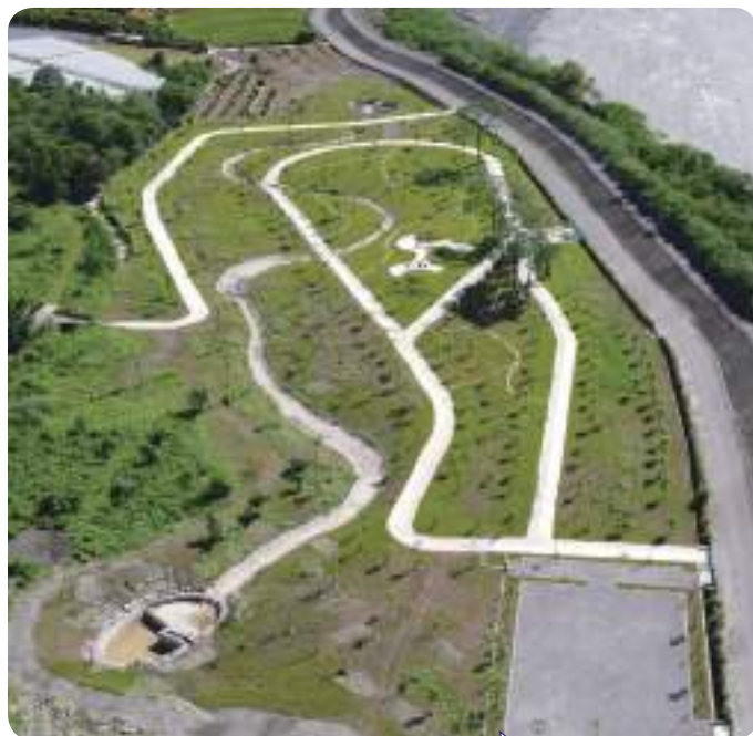
十八羅漢山自行車服務中心週邊環境改善工程 Eighteen Arhats Mountain Bicycle Service Center Surrounding Environment Improvement Project
