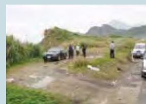
▲台2線73k+800—施工前
