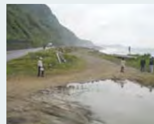
▲台2線80k+500水溝洞—施工前
